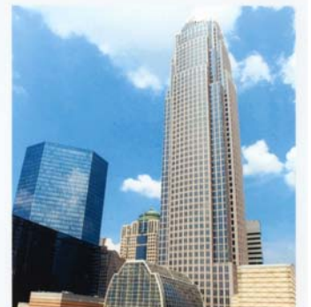
BANK OF AMERICA CORPORATE CENTER Charlotte, N.C. Completed: 1992
