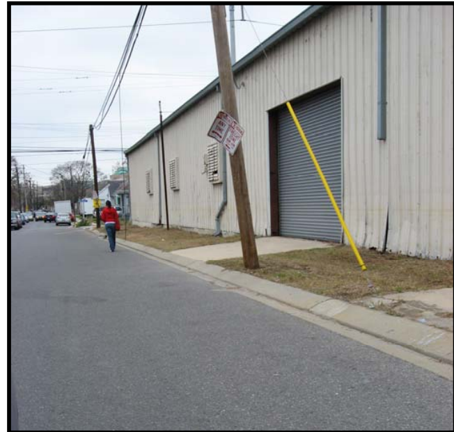
Photo 1- Lack of sidewalk along Dixon Street
