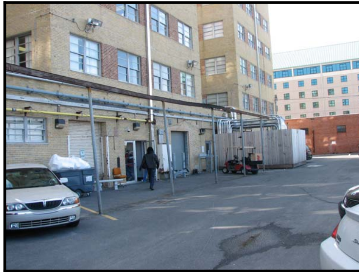
Photo 4- Xavier South service entrance
