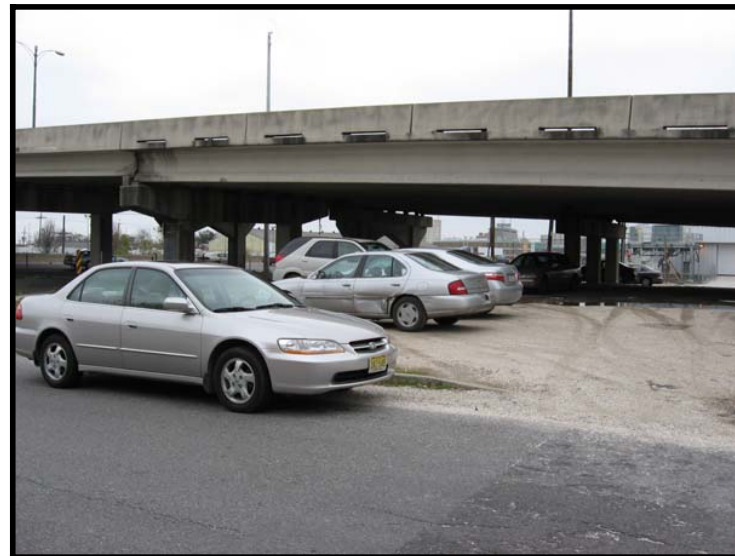
Photo 6 – Parking underneath the Jefferson Davis Parkway Overpass
