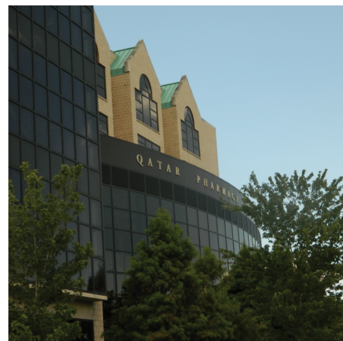
SIGNATURE BUILDING SIGNAGE
