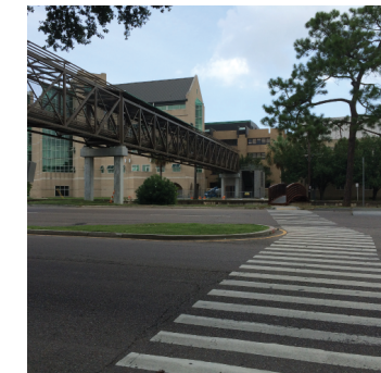
3 PEDESTRIAN BRIDGE OVER CANAL
